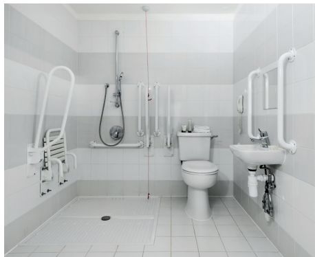
The designated accessible bedroom has a wet room with a left-hand transfer lavatory. There are 3 grab bars around the lavatory, one is retracting. The third is not shown and is horizontal to lavatory (obscured by sink in this image). There is a handheld and ceiling shower and 2 vertical grab bars, one retracting and 1 horizontal. There are 2 wall mounted shower chairs (2nd is out of view on left of image). The floors and walls have white tiles with pale grey tiles as a border to the floor and a 2nd border highlights location of the grab bars. The emergency cord will reach the floor.
